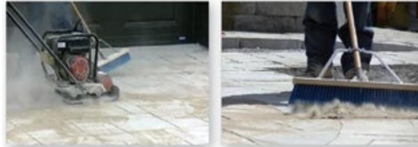
**STEP 4:** To ensure that no sand sticks to the surface of the pavers, use a stiff bristled broom for the initial sweeping of the polymeric sand. Then use a soft bristle broom to sweep the excess sand off the surface. Finally, use a leaf blower to ensure the removal of any excess sand residue from the surface. These two cleaning steps are important before proceeding to step 5.
